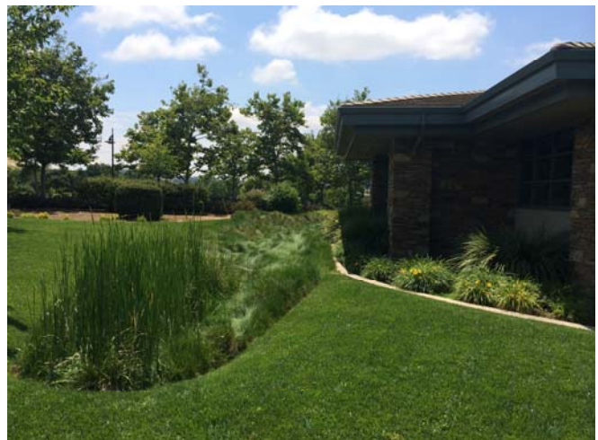
Backyard swale at County of El Dorado Facility
